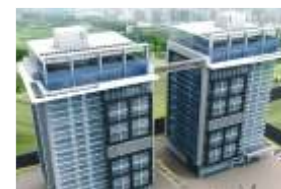
UDB Corporate Towers
